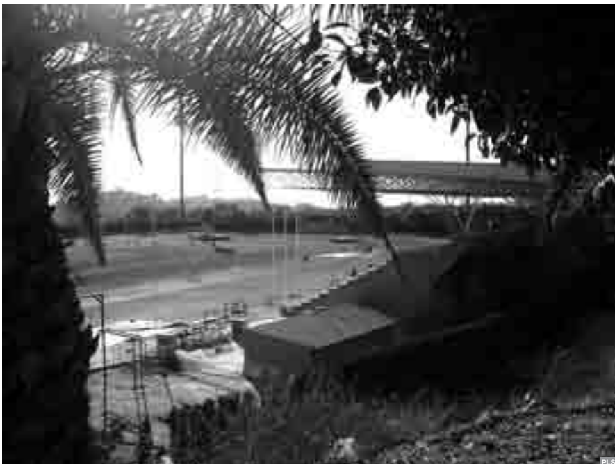
▲ Panoramic view of the Athletics Stadium «Monte Romero», in whose interior a fitness room is located.
